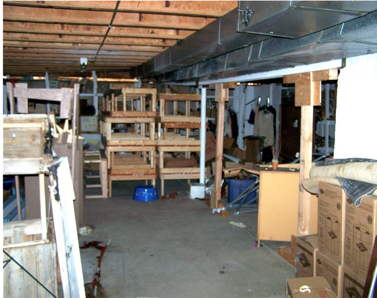
GB _ Church Damage -2
